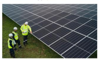
Solar energy parks use interconnected photovoltaic panels to capture sunlight, creating DC electricity which is then converted to AC by on-site invertors. Solar power is a renewable and infinite resource.
