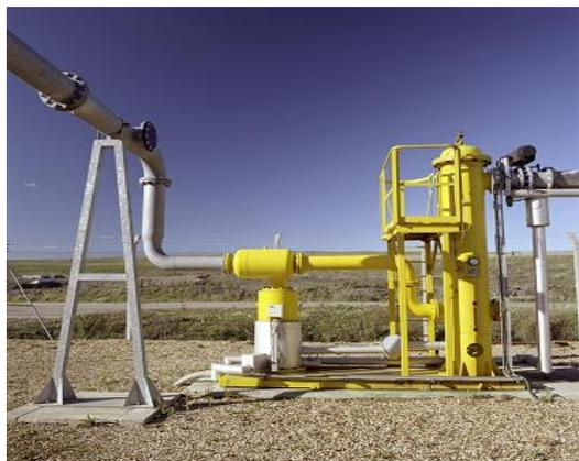
Gas de-watering and filtration plant for Brogborough phase V landfill gas generators
