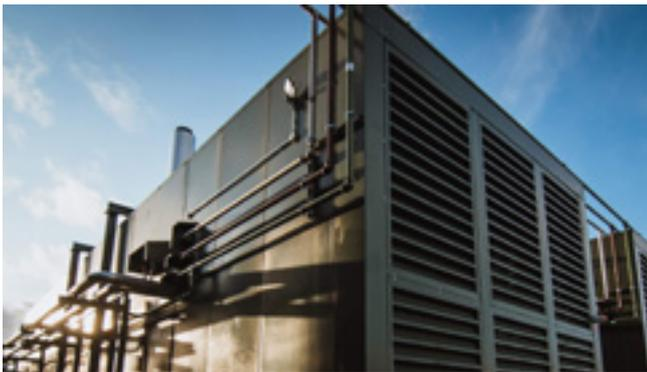
Power Response (PR) provides highly responsive power in local areas connected through the local distribution network closest to consumer demand, using mostly mains natural gas to power modular gas reciprocating engines. PR supports the UK's energy transition and growing intermittent renewable power generation, from wind and solar, whilst also providing back up capacity in the event of grid demand.
